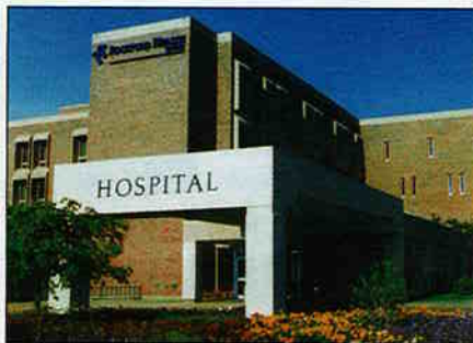
Rockford Memorial Hospital in Rockford, IL performs 10,000 surgical procedures per year.
